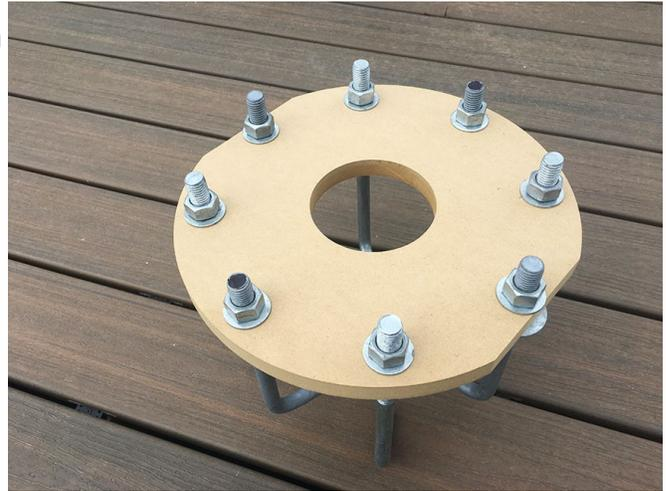
around the bolts. Level the template in the north-south and east-west directions. If the concrete has not yet set enough to hold the bolt location, check the level every 10 minutes until the template no longer moves. You may also use blocks and shims attached to the forms to hold the template in place. Insure that all bolts are plumb. If bolts are not cast plumb, the pier might not slide easily over the bolts.
